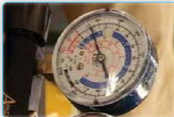
Refrigerant pressure displayed on the recovery gauge
