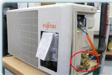
Split system air conditioner access ports
