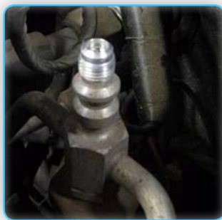
R12 access point
