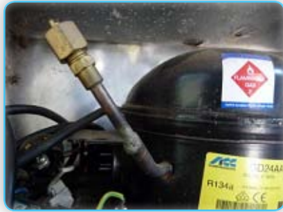
Process tube with Schrader valve
