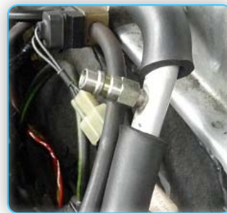
R134a access point
