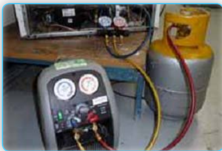
Refrigerant recovery unit and service hose setup
