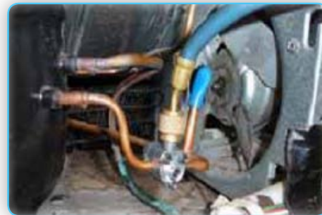
Bullet valve clamped on pipe
